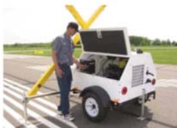
4. Start the generator and activate the lights
