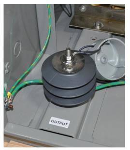
Figure 6: Output Surge Arrestor without cap
