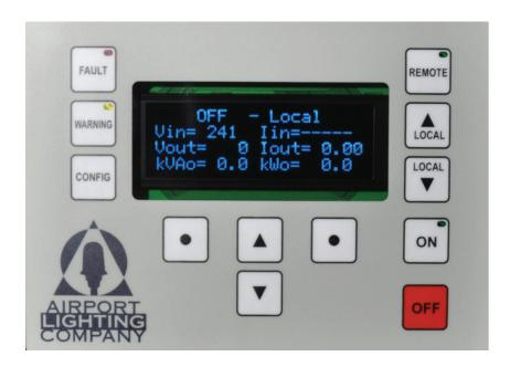
Figure 11: Keypad and Display of a 240V input CCR
