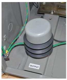
Figure 5: Output Surge Arrestor with cap
