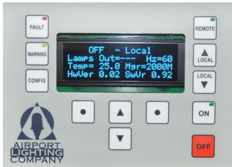
Figure 14: Megger Measurement (Open Circuit)
