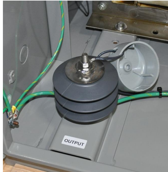
Figure 7: Output Surge Arrestor without cap
