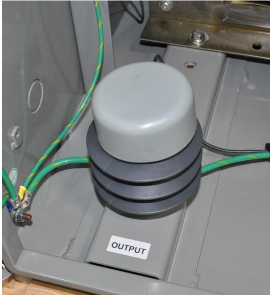
Figure 6: Output Surge Arrestor with cap
